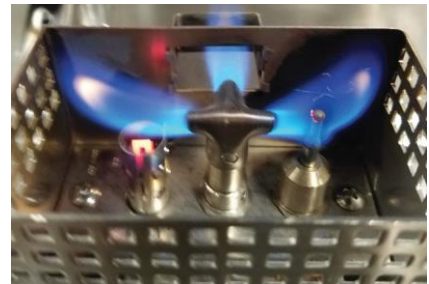
Figure 9.2 – Pilot flame coverage of thermocouple.
