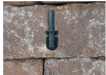
Figure 6.8 – Dry fit the bracket
