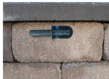
Figure 6.5 – Fasten down the bracket
