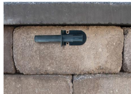
Figure 6.4 – Dry fit the bracket
