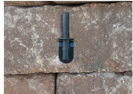
Figure 6.9 – Fasten down the bracket
