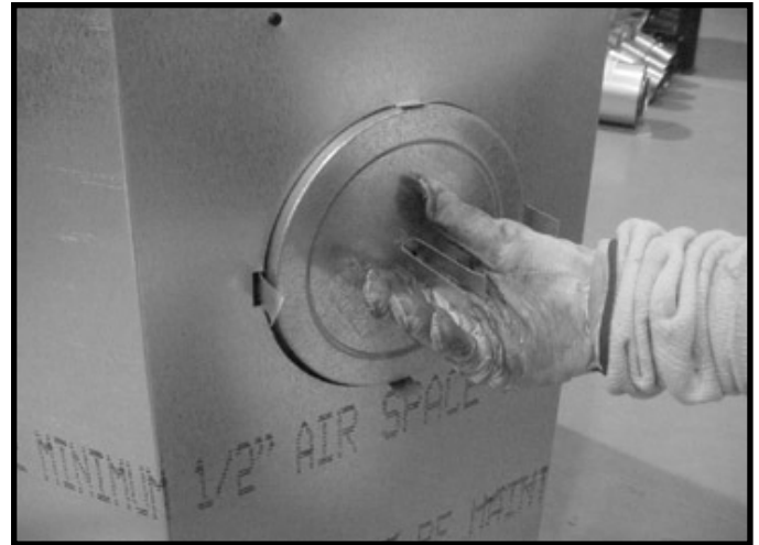
Figure 6.8 (Generic Fireplace Shown) Fold the center parts of the retaining band out and use to remove the seal cap.
