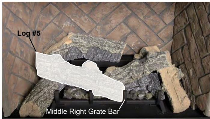
Step 6: Place the end of Log #5 against middle right Grate Bar as shown. The other end will rest on Log #2.
