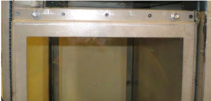
Top of Glass Door Frame
